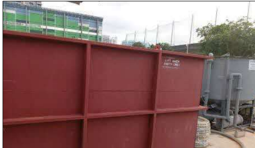
Additional Storage Tank (12m3)
