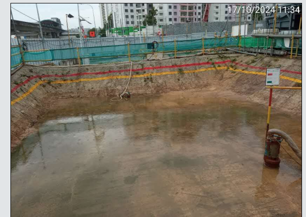
Collection pond & sprinkler pump
